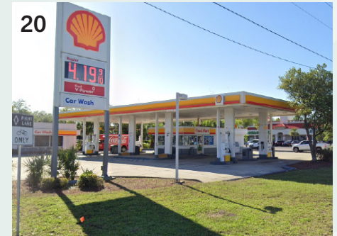
10716 Atlantic Blvd, Jacksonville, FL
